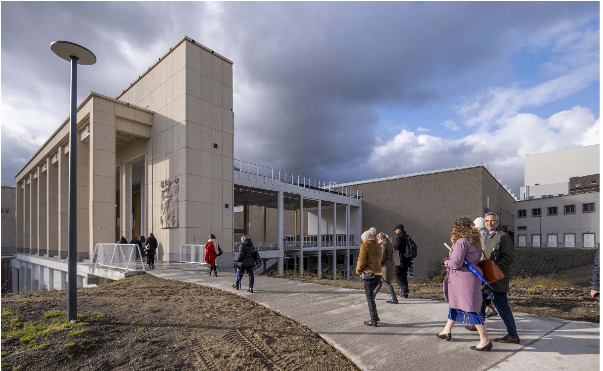
Visit of the Charleroi Great Palace, renovation designed by architecten de vylder vinck taillieu in association with AgwA, appointed in the framework of the assistance provided by the Charleroi Bouwmeester.
