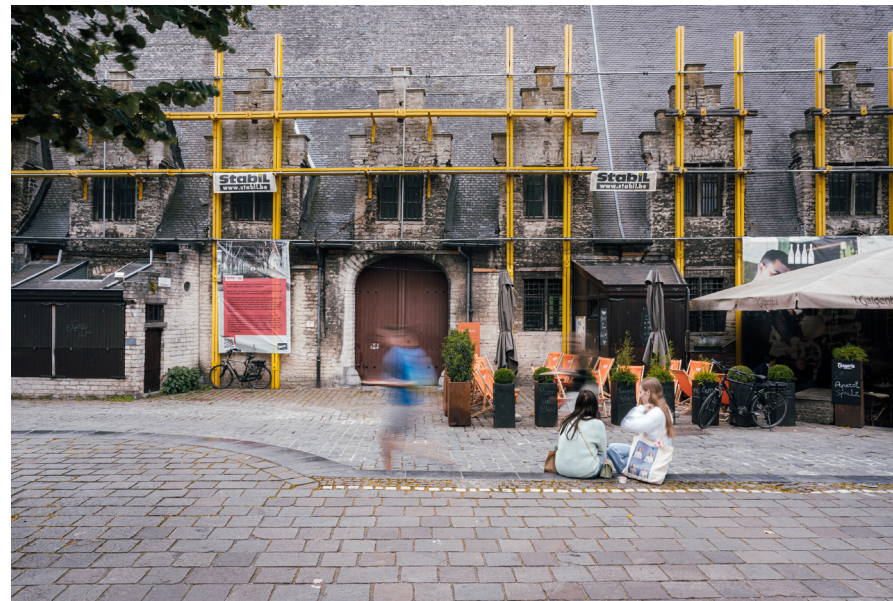
fig.3 Great Butchers Hall in scaffolding © City of Ghent, photo: Rosan Steenbrugge
